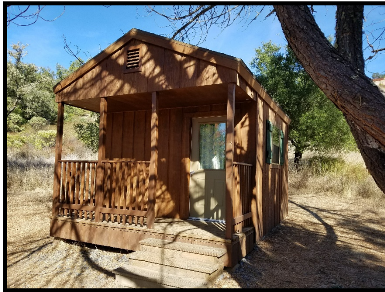
Figure 32 - Example of Improved Camping Facility at Lake Sonoma
